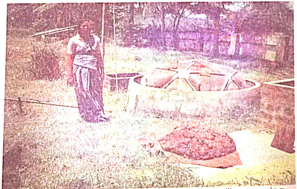
A domestic biogas digester in an Indian village, using animal manure and producing methane for cooking and heating water.
